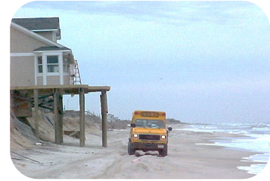
Flooding and Erosion Hazards
